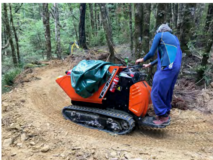
Compacting the surface with the powerbarrow
