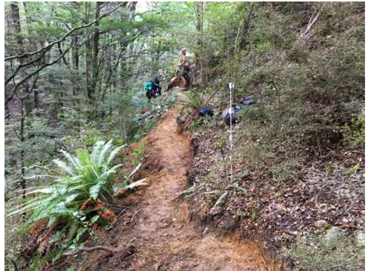
Hand building the steep gully on Lowther Link
